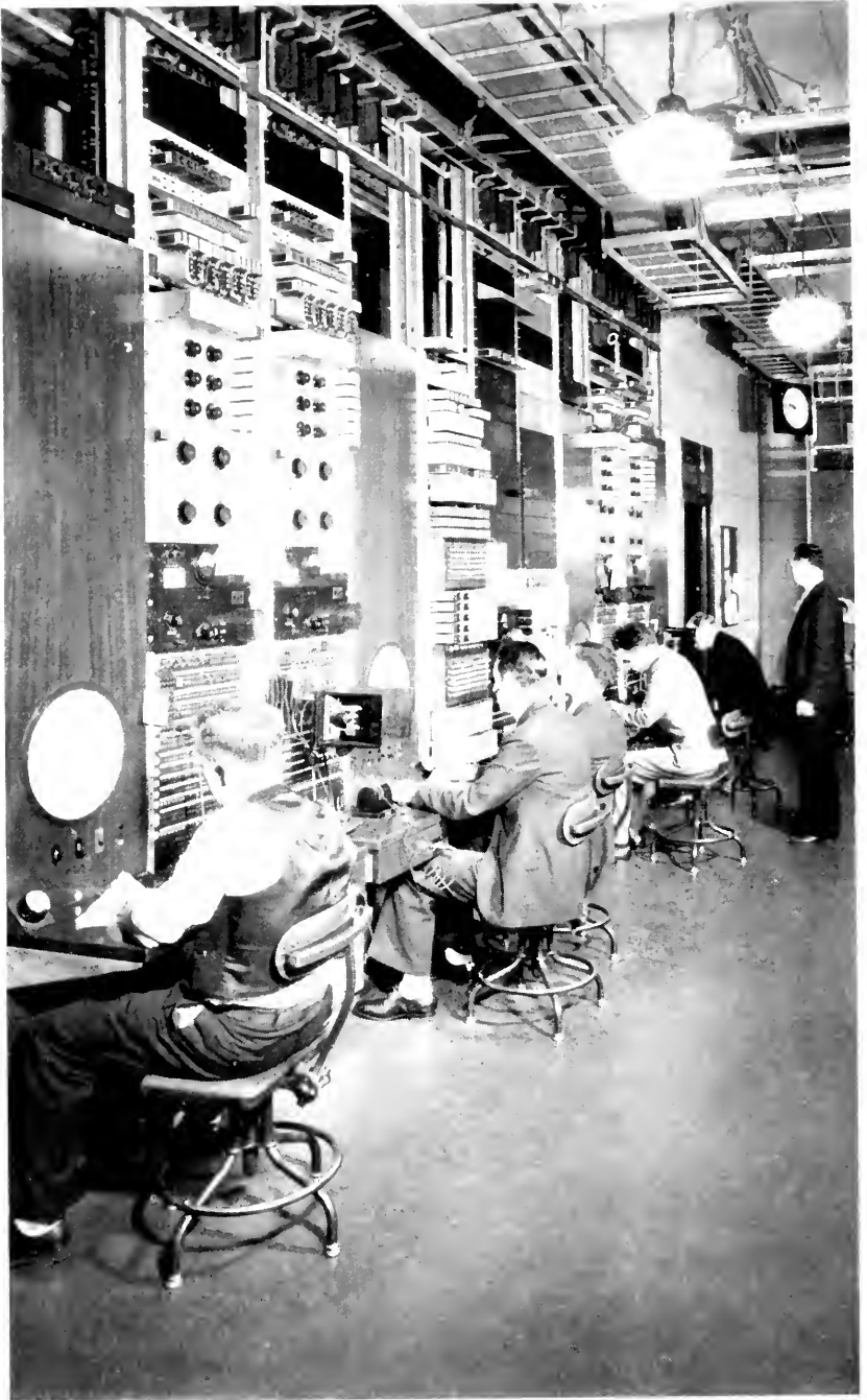
A SECTION OF THE TELEPHONE COMPANY'S MAIN SWITCHING OFFICE IN CHICAGO. Here, in the course of a week, as many as 600 switching operations take place in routing radio programs, as explained in the article which begins on the opposite page.
